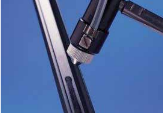
Spraying activator onto window trim
